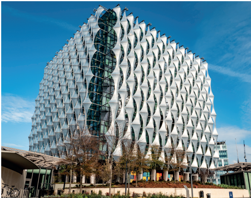
A view of the exterior of the new US Embassy in the Nine Elms (Wandsworth) area of South West London
